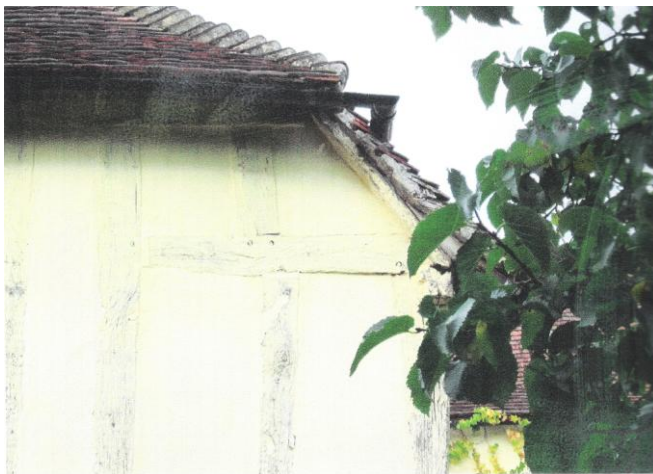
Photo 21: Half-timbering at Paycocke's
